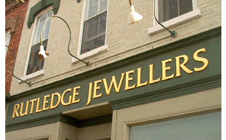
Figure 20 When storefront signage is located on the entablature above the storefront, opportunities for traditional lighting exist.
