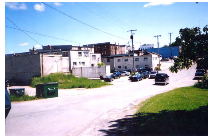
Figure 70 Back lot views off Albert Street to buildings fronting onto Brock Street.
