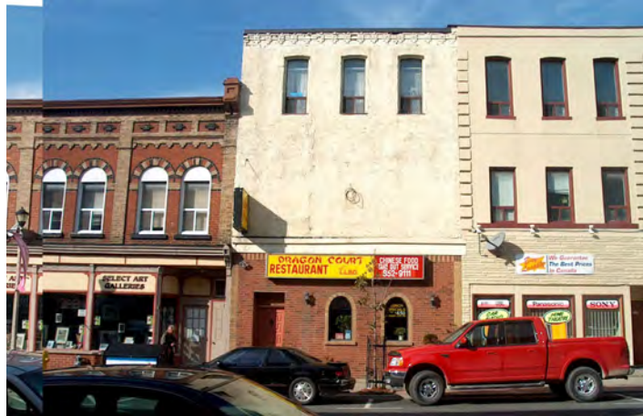
Figure 18 It appears from a cursory inspection of the building in the middle that window openings still exist behind the stucco cladding and could be re-opened without too much difficulty.
