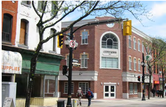
Figure 40 This example of a contemporary corner building takes full advantage of its corner location and frontage on two streets.
