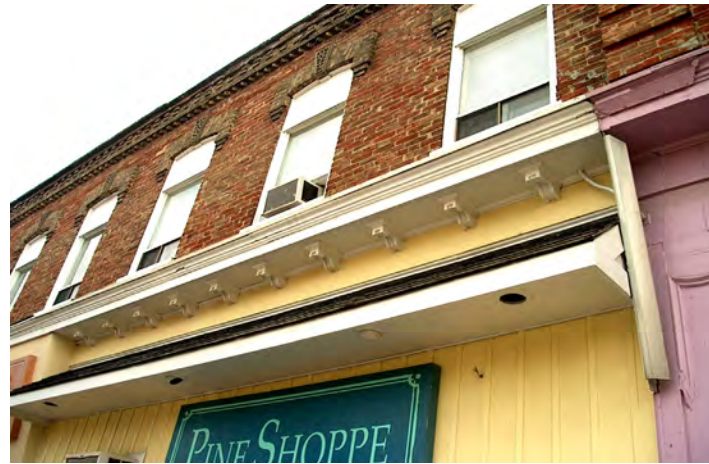
Figure 15 In many cases the heritage façade still exists behind modifications made to the storefront assembly over the years. Lowe's Furniture Store may well be an example of this.
