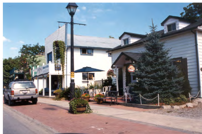
Figure 63 This widened boulevard and setback in Kleinburg accommodates off street parking and a generous sidewalk.
