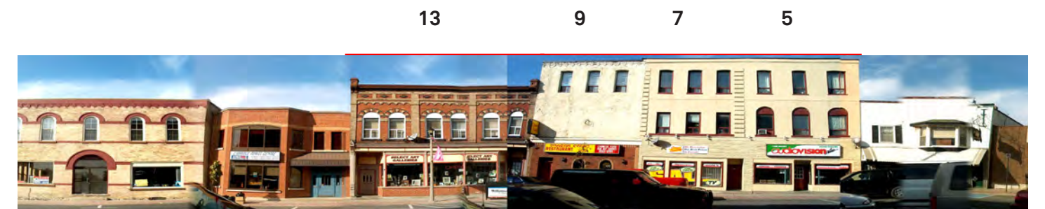
Figure 6 The Art Shop located at 13 Brock Street is a fine example of what can be accomplished through careful and thoughtful restoration. The buildings immediately to its east (9, 7, and 5 Brock Street) are excellent candidates for this same level of treatment.
