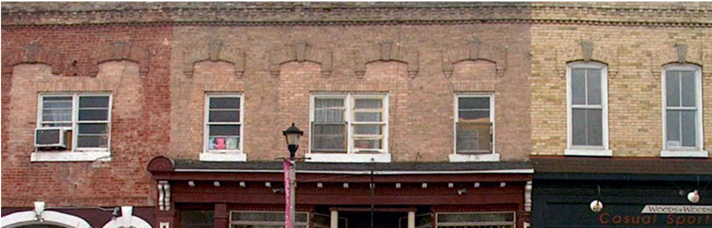
Figure 19 In situations where the original windows have been removed and window openings filled in, consult a restoration architect or a heritage contractor prior to breaking open the masonry mass.
