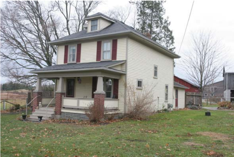
Plate 5: Looking southwest at existing residential structure; HI immediately north of this house
