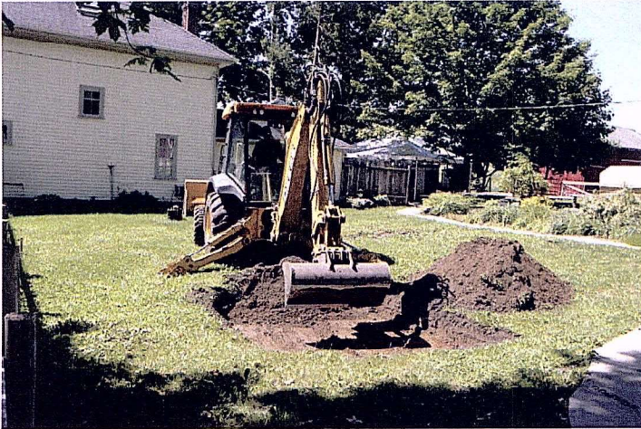
Plate 7: View of the Stage 4 striping of topsoil at the northwest portion of the Charlie Site
