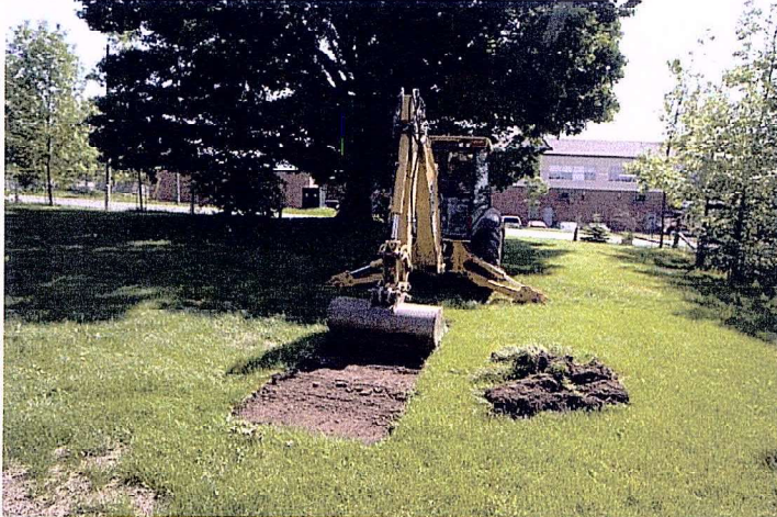
Plate 4: View of the Stage 4 striping of topsoil at the northeast portion of the Charlie Site
