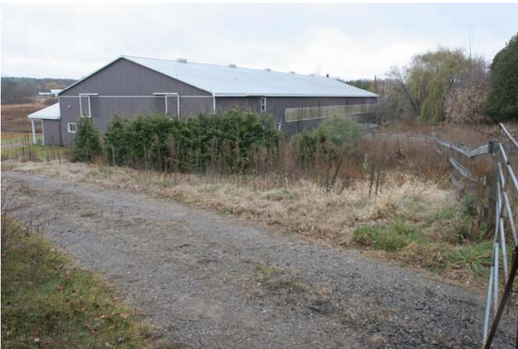
Plate 6: Looking southwest at gravel driveway and barn structure
