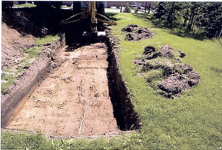
Plate 5: Close-up view of the Stage 4 striping of topsoil at the northeast portion of the Charlie Site
