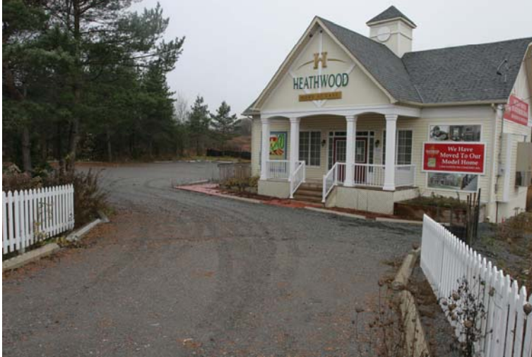
Plate 1: Looking south at existing sales centre and gravel driveway
