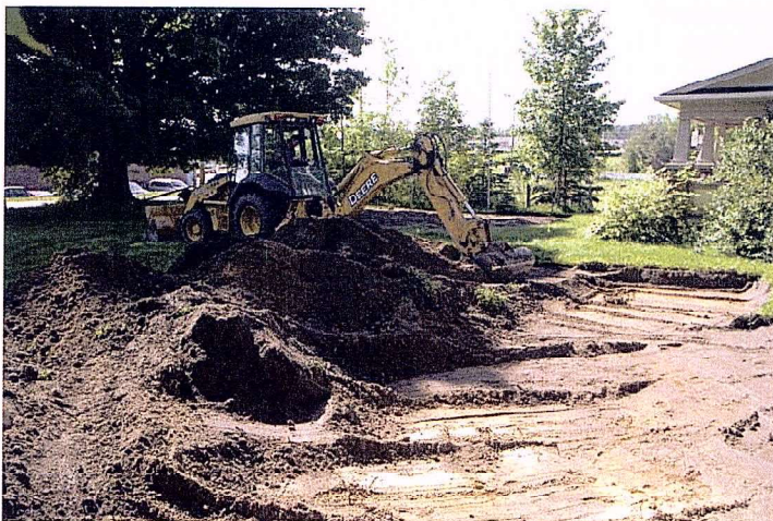
Plate 6: View of the Stage 4 striping of topsoil at the northeast portion of the Charlie Site
