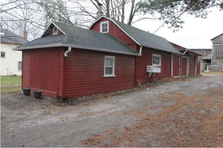
Plate 4: Looking southwest at existing structures on site
