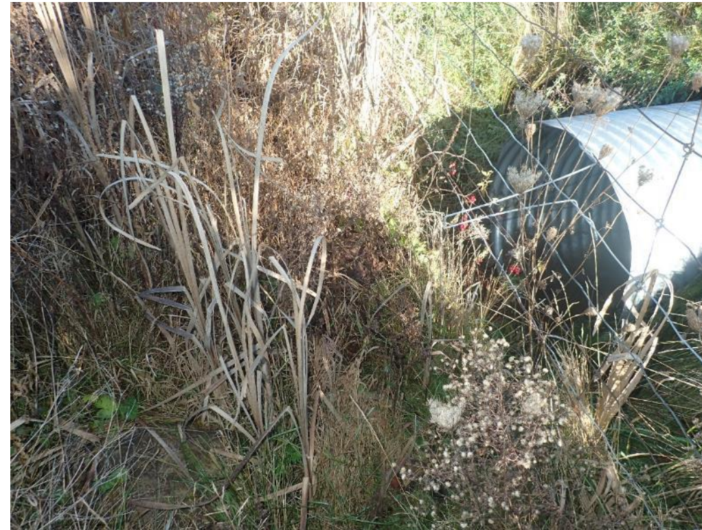
Image 10 View of disturbance associated with culvert.
