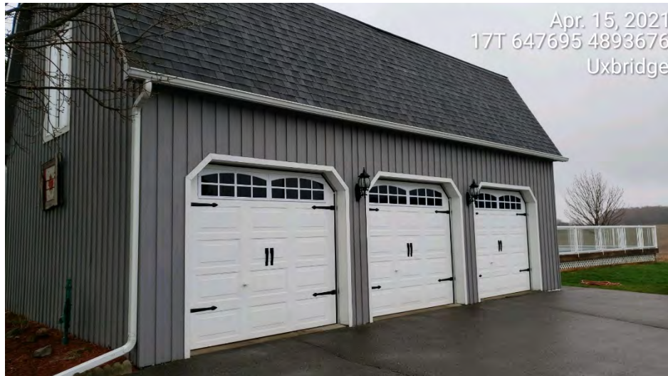
Photo 3 – Drive shed / garage.
