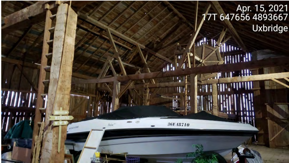
Photo 6 – Storage within the barn.
