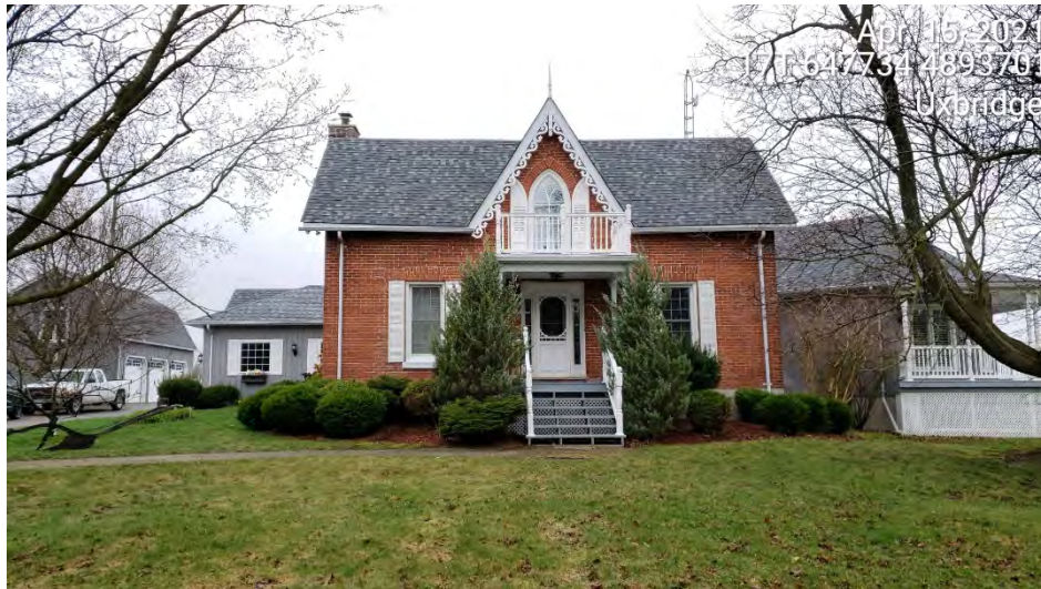
Photo 1 – Existing residence at 10700 Regional Road 1 in Uxbridge.
