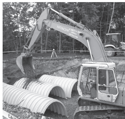
No equipment shall be operated on the bed at this stage of the installation. Excavators must be located off the bed. Dump trucks shall not dump stone directly on to the bed. Dozers or loaders are not allowed on the bed at this time.
