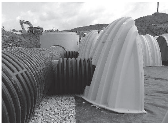
Align the first chamber and end cap of each row with inlet pipes. Contractor may choose to postpone stone placement around end chambers and leave ends of rows open for easy inspection of chambers during the backfill process.
