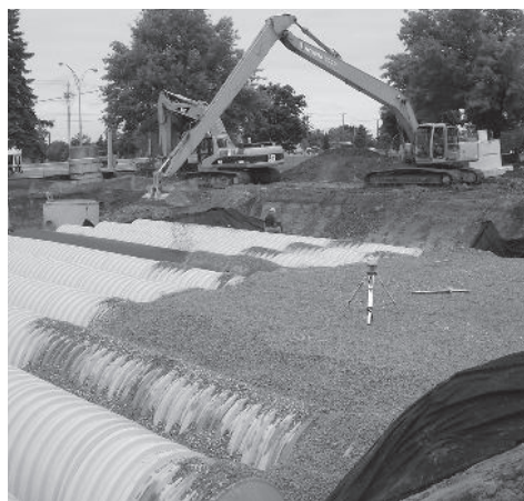
No equipment shall be operated on the bed at this stage of the installation. Excavators must be located off the bed. Dump trucks shall not dump stone directly on to the bed. Dozers or loaders are not allowed on the bed at this time.
