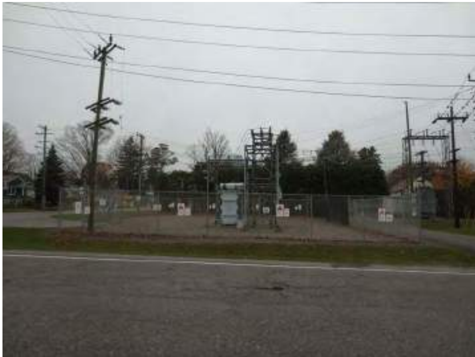
Photo 13 – Neighbouring land to the west: electrical substation (looking west across Donland Lane).
