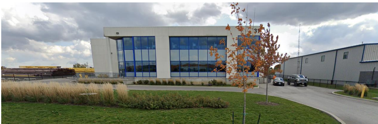
FIGURE 5 – SOUTH ADJACENT COMMERCIAL BUILDING
