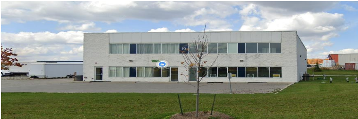
FIGURE 4 – EAST ADJACENT COMMERCIAL BUILDING
