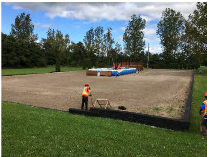
Photo 12: View of dog training area with sand pit, dock structure and pool – looking northeast
