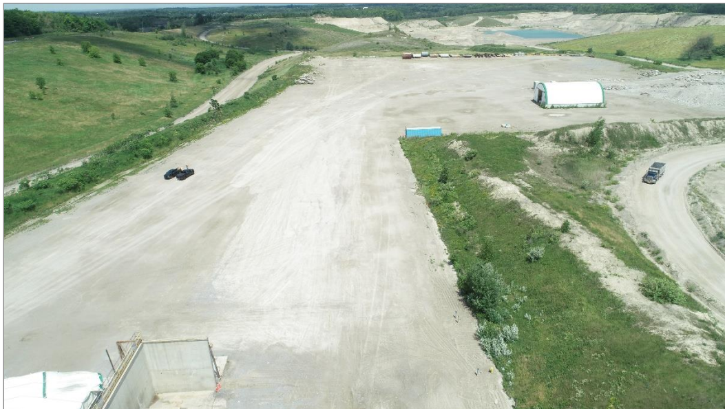
Figure 2.7 Looking north from centre of the site (existing finishing tent in the top right)
