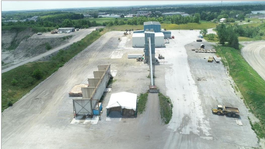
Figure 2.6 Looking south over centre of site (aggregate storage and conveyor in foreground)
