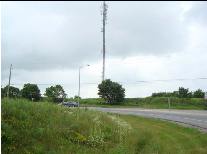
Communications tower east of subject property, looking east
