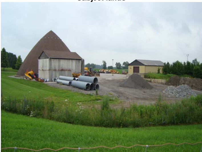
Region of Durham Works Department, Scugog Depot, southeast of subject lands
