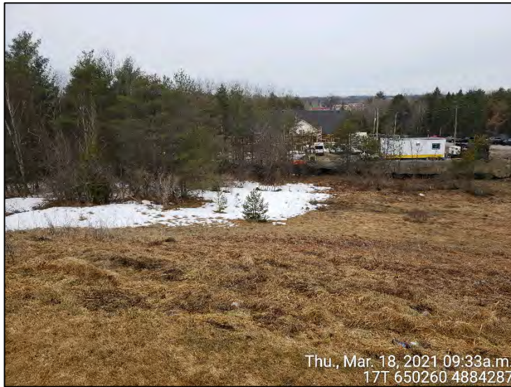
Photo 2 - View from parking lot area towards adjacent new residential construction.
