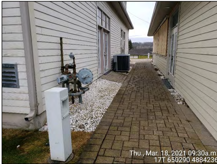
Photo 6 - Clubhouse building is heated with natural gas.
