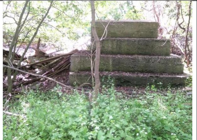
IMAGE 4 CONCRETE AND STONE FOUNDATION
