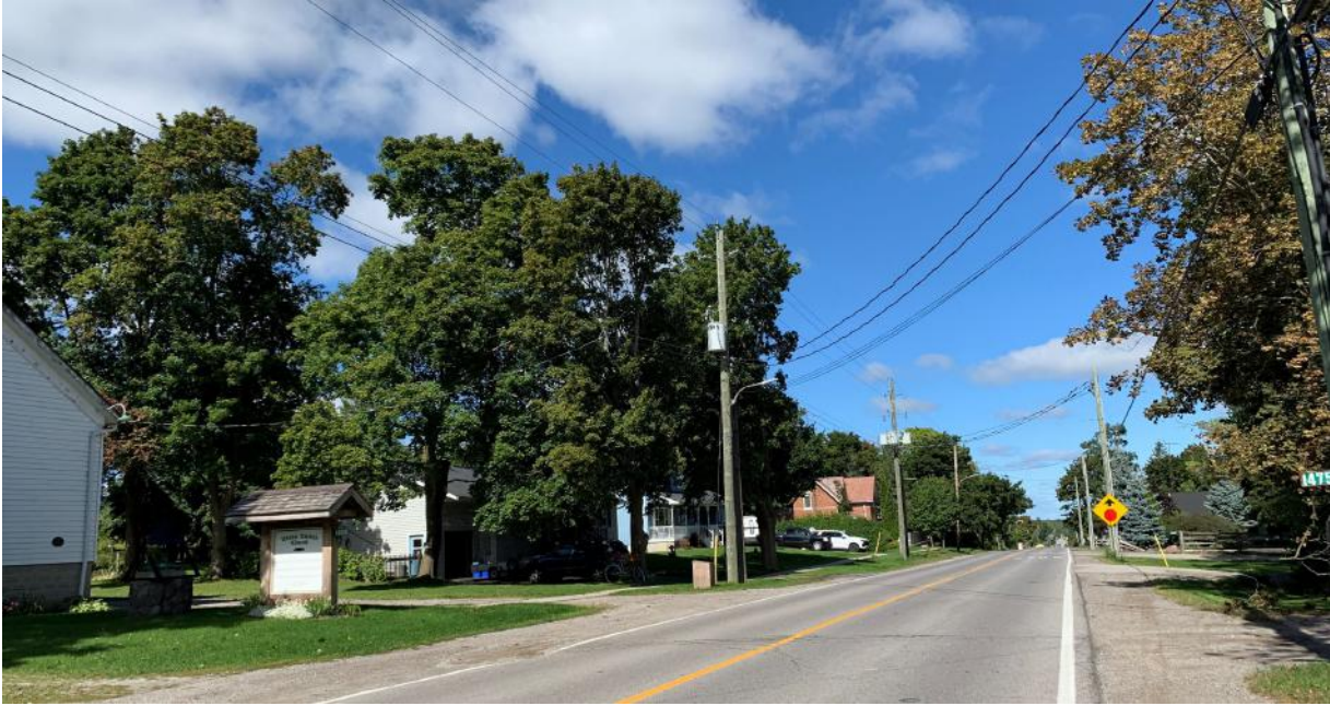
Photo 9 View of Regional Road 1, facing north
