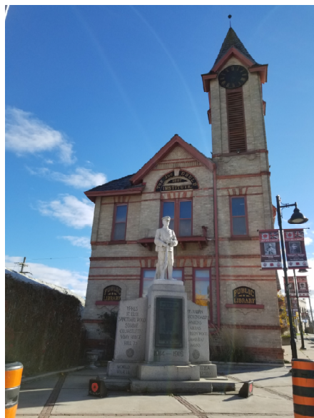
Fig 7 – Existing Uxbridge Masonry Fabric
