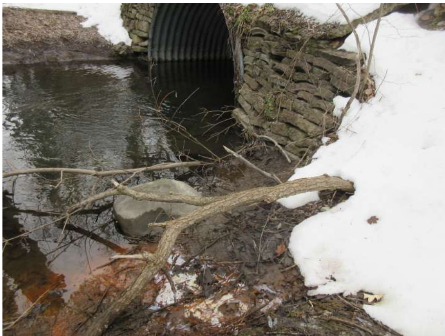
PHOTOGRAPH 3: Orange/rust staining along creek bank, upstream of outfall, ground water discharge location
