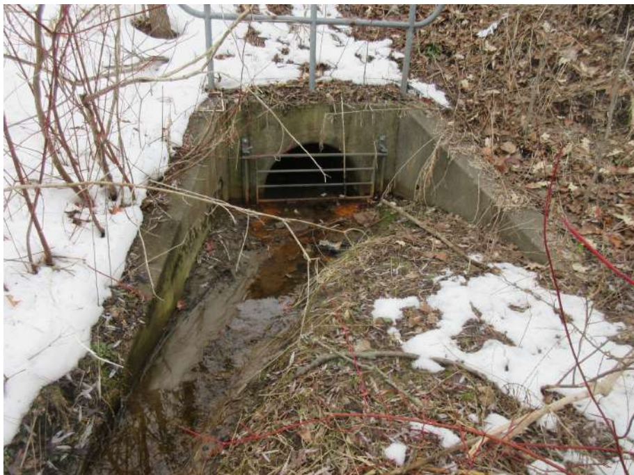
PHOTOGRAPH 2: Poplar Street outfall, note orange/rust staining
