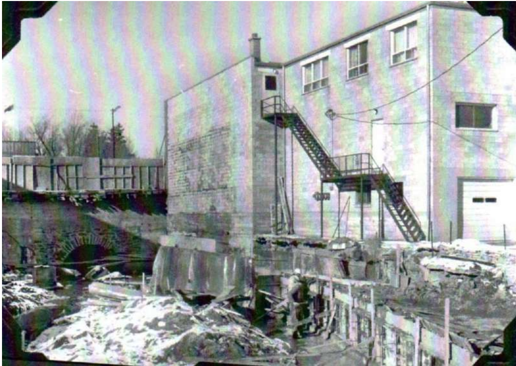
Image 3: Looking north at construction activities during installation of culvert immediately south of Brock Street, November 1972. The building to the right still exists today (see Image 6) (Courtesy of Uxbridge Public Library)
